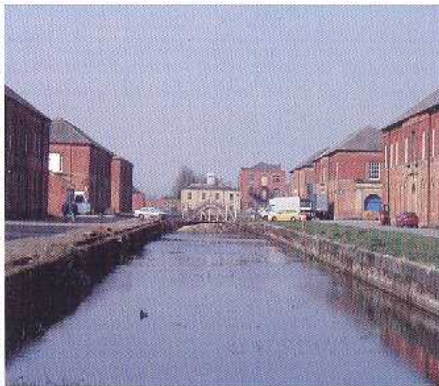
An impressive view. The Museum site being prepared for the long awaited opening in 2003.
